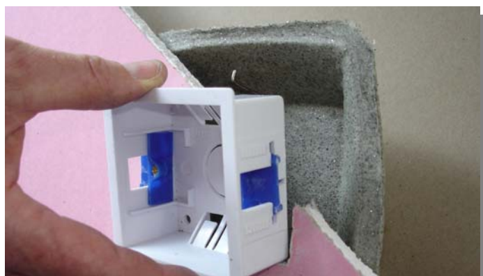
Installation of box
