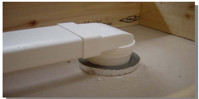
Fan Firecap CFS100 with Flat Ducting
